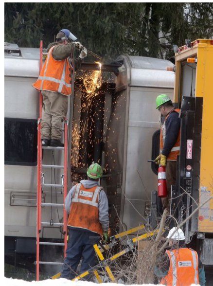
The third rail punctured the Metro-North train’s first car and ended up near the roof and between the first and second cars after the Tuesday evening crash. A portion of third rail is cut Wednesday as workers begin the process of removing the wreckage. (Photo: Seth Harrison/The Journal News)
