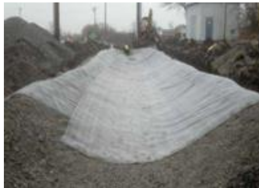
Reactive Core Mat Installation
