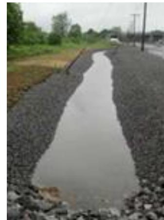
Restored Drainage Ditch
