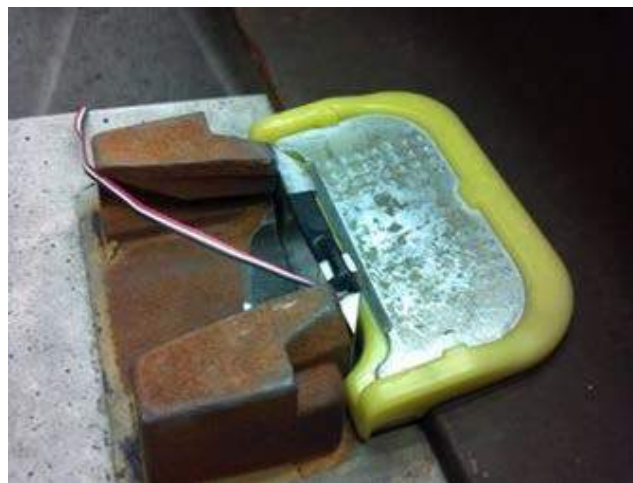
Figure 26. LLED Installation Prior to Clip Application
