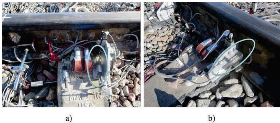
Figure 242. Linear Potentiometers Installed to Measure a) Rail Base Lateral Displacement and b) Rail Web Lateral Displacement
