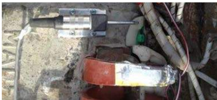
Figure 28. Lateral Rail Pad Assembly Displacement
