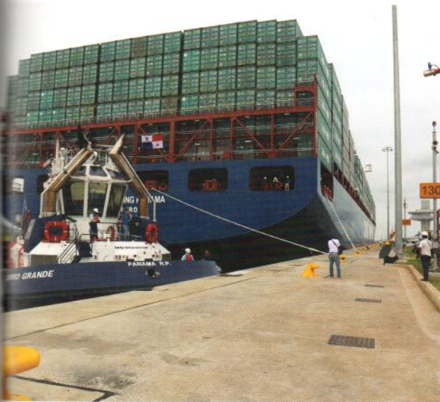
In 2016 the Marine Board and Marine Group activities focused on infrastructure needs from the larger ships crossing the newly expanded Panama Canal. (Photo: U.S. Embassy Panama)
