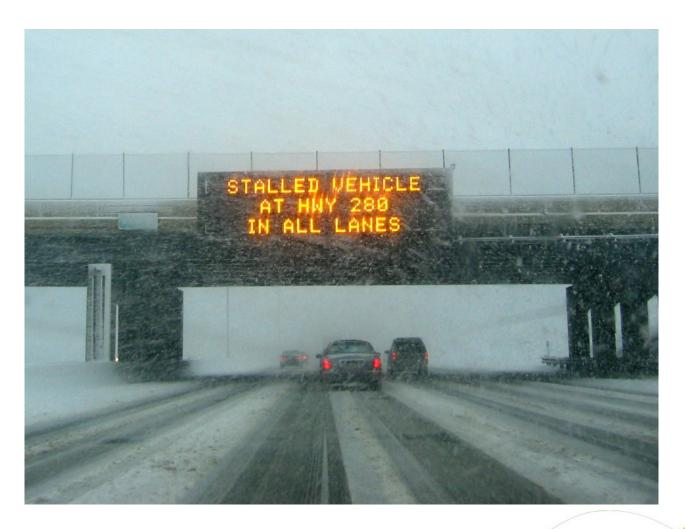
Image of a variable message sign, could be applied to notify road users of time of occupied crossing to reduce risky behavior
