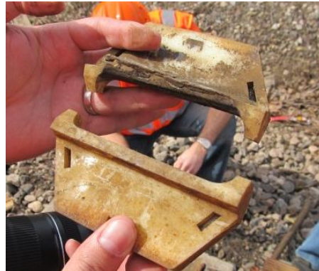
Insulator post wear
