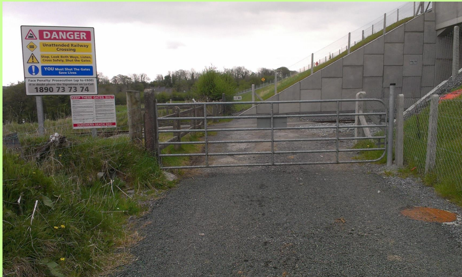
Grade separated closure of passive road level crossing
