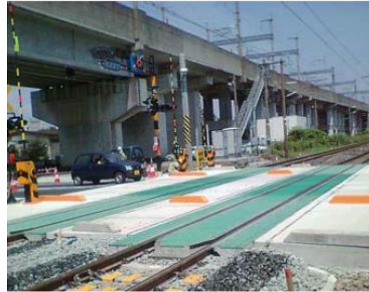
Precast prestressed crossing
