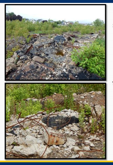
The vacant site contained large piles of debris and concrete rubble from the demolition of the former buildings, as well as the concrete footers and foundations.
