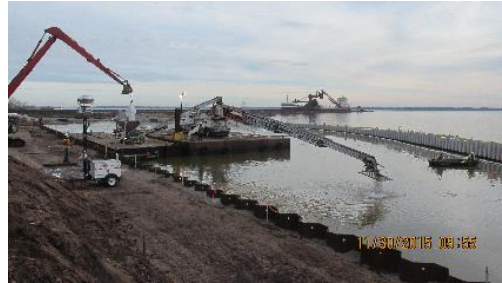
Granular Bentonite Placement
