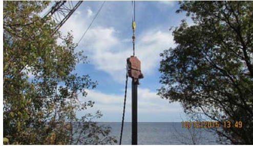
Vibratory Hammer Used to Install Sheet Piles
