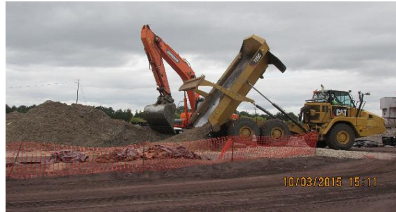
Dredge Spoils Loaded in Dewatering Area
