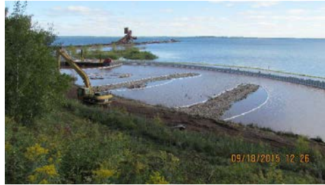
Finger Piers Constructed for Access
