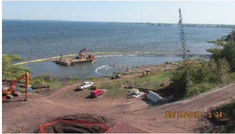
Installing Temporary Perimeter Sheet Pile Wall
