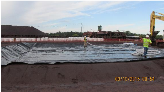
Dewatering Pad Constructed
