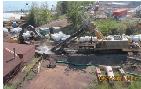
Bulk Bentonite Added For Lubrication
