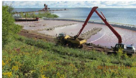
Loading Spoils for Transport To Dewatering Area
