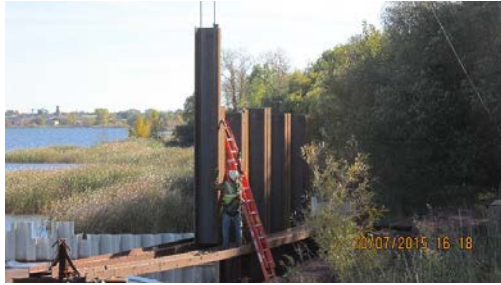
Sheet Pile Setup on Shoreline
