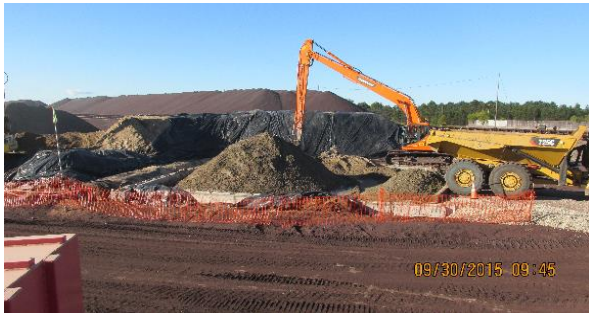
Dredge Spoils Dewatering
