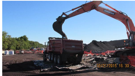
After Dewatering, Sediment Loaded for Offsite Disposal
