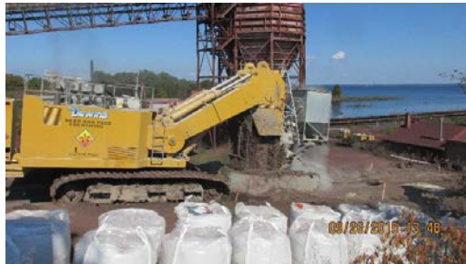
Bulk Bentonite Metered into Trench
