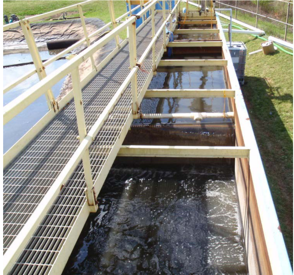
Rectangular Steel "Frac" Tanks
