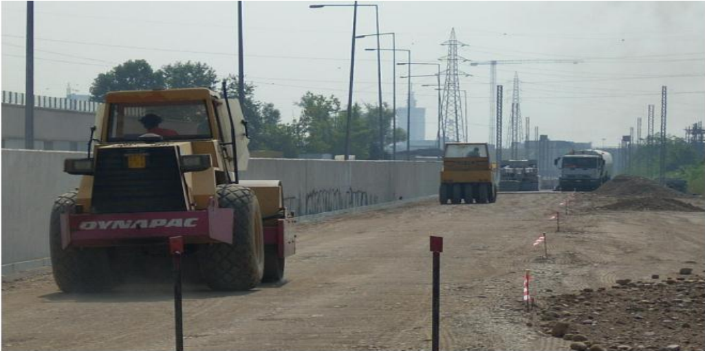
Compacting Subgrade and Placing/Compacting Asphalt
