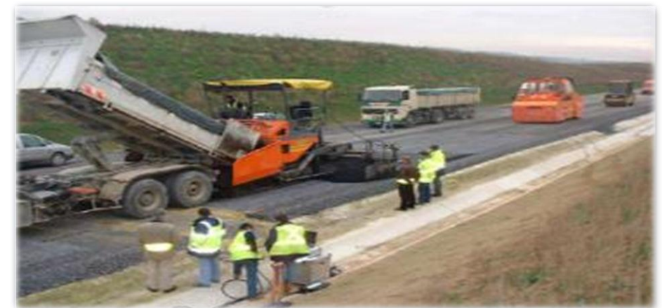
Construction of the test area - layer of pervious
