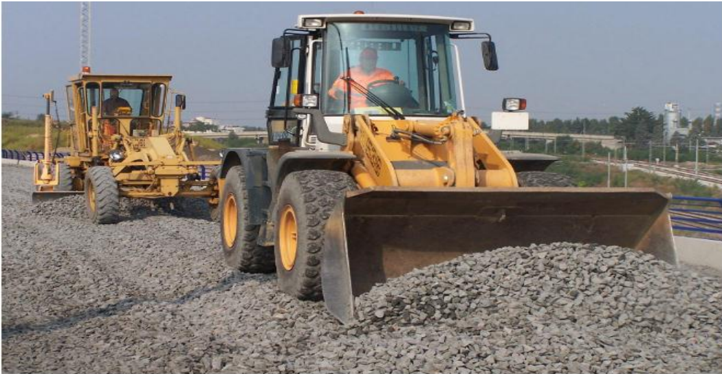
Spreading and Compacting Ballast
