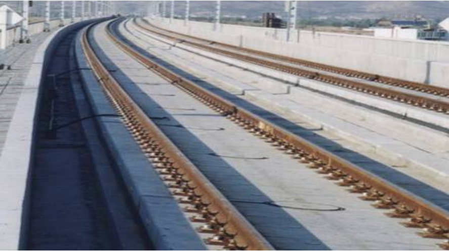
CRTS I SLAB
