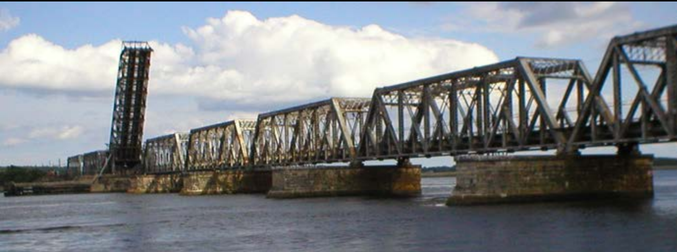
Connecticut River Bridge, Hardesty & Hanover ( http://bit.ly/1LJ82Ek ).
