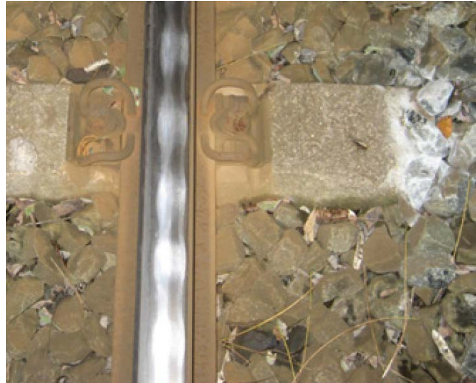
short-pitch corrugation (Source: Correa, 2011)
