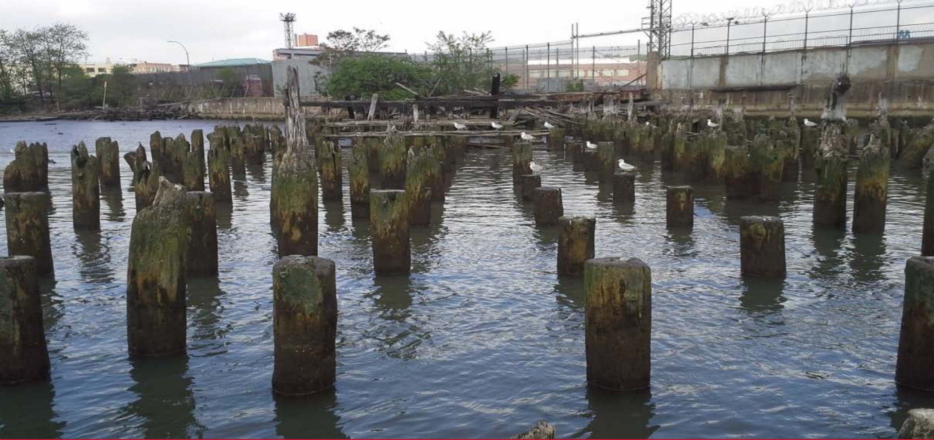
Timber Pier Perch Habitat
