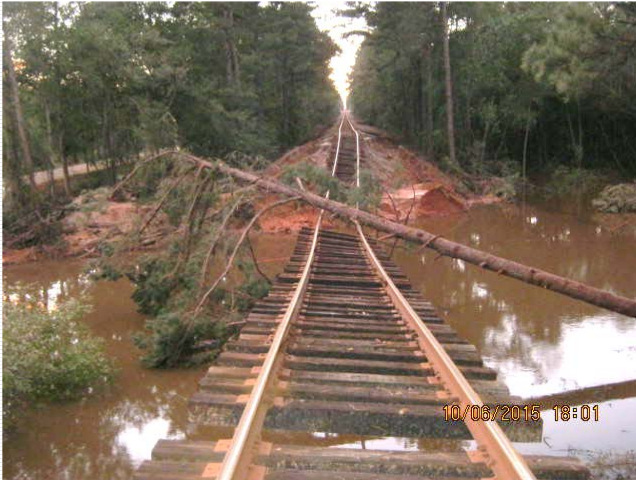
AKA 360.3 – 12' Brick Arch at Cedar Creek
