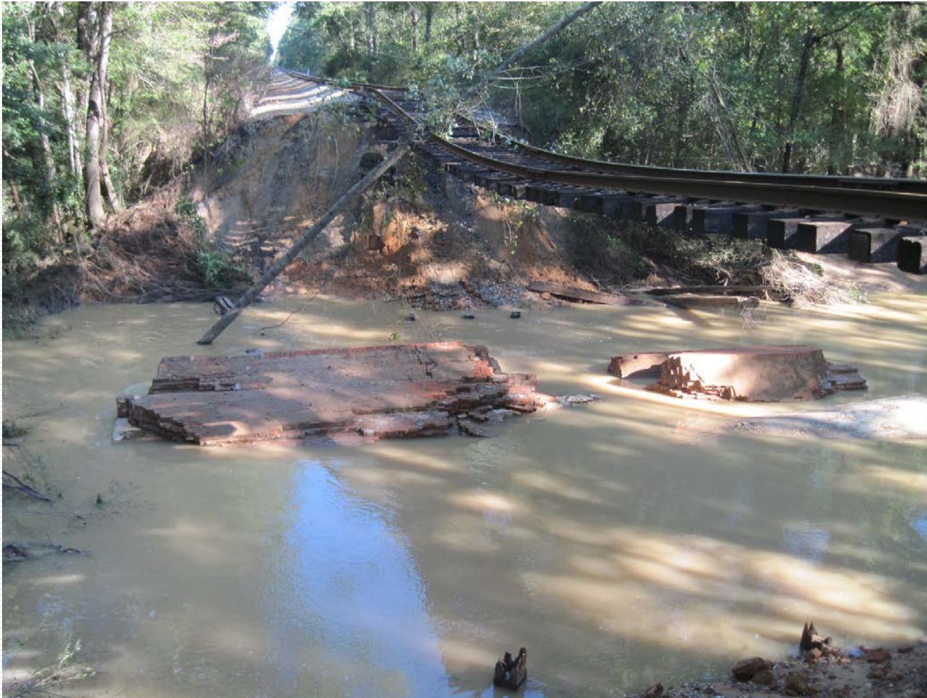
AKA 366.1 – 10' Brick Arch at Mill Creek
