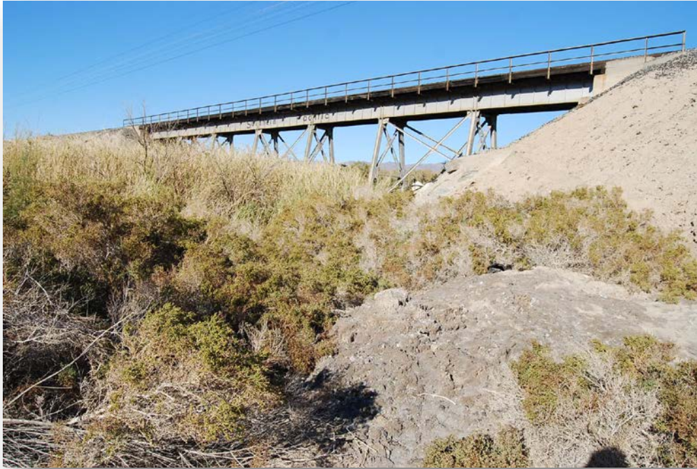
Existing bridge at Salt Creek, Riverside County, California
