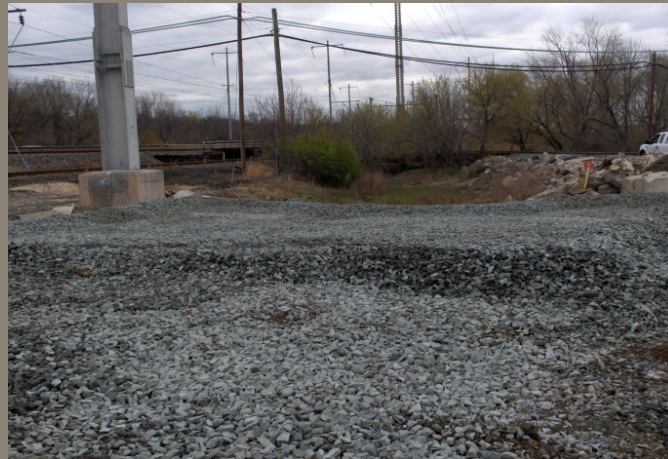
Localized E&S Controls
