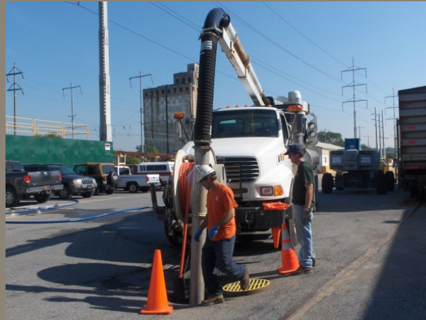
Outfall 002 Storm Sewer Cleanout
