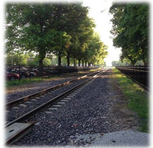
Right-of-way fencing installed within urban areas within Union Pacific Railroad ROW
