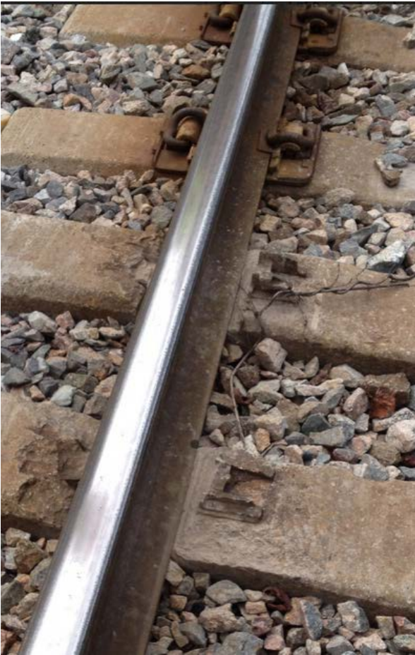
Broken/Worn Shoulder
