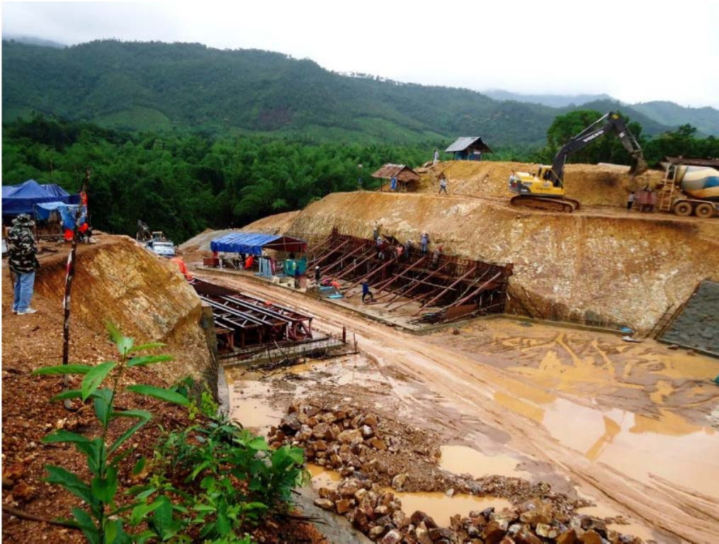
Dam Construction: Transition Wall and Slap Casted Progress (Source: ITD, 2013).
