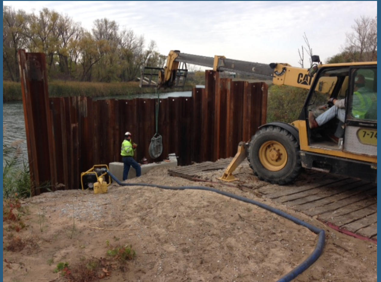
Installation of the flap gate on the outfall headwall
