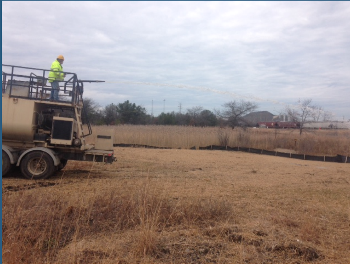
Hydro-seeding and mulching temporary cover crop
