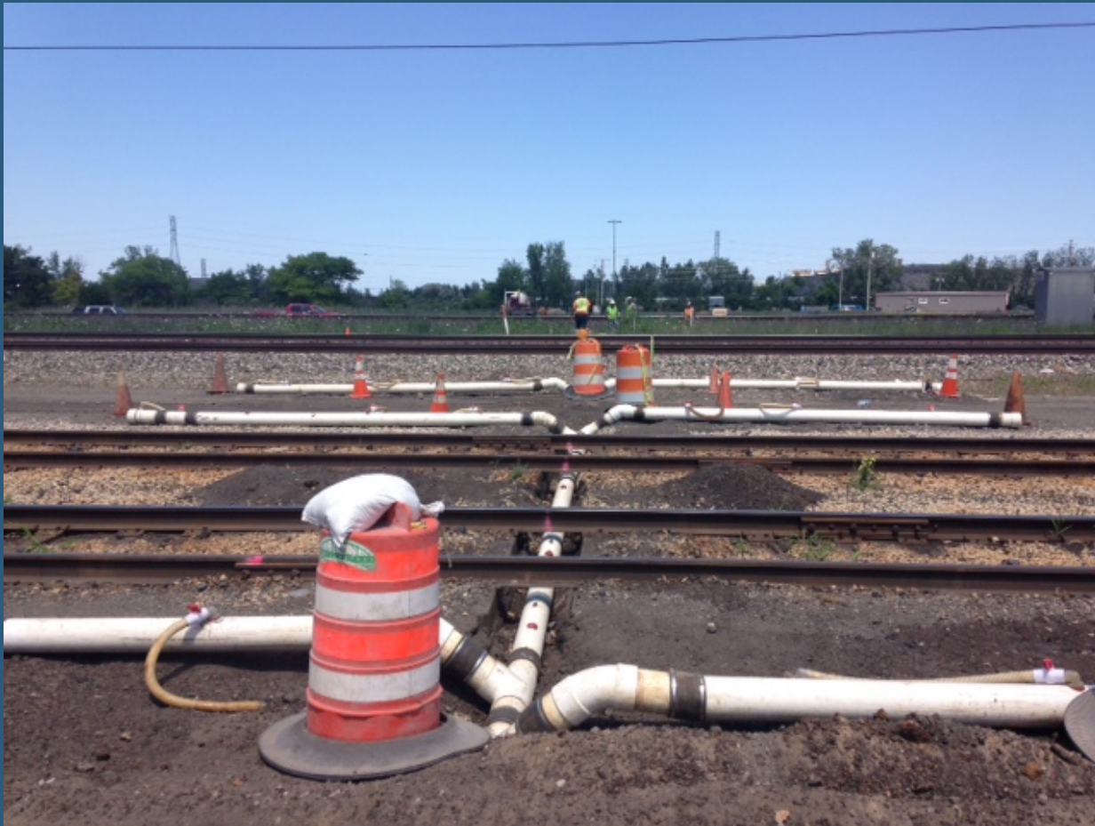
Dewatering along pipe alignment to prevent running sand during bore
