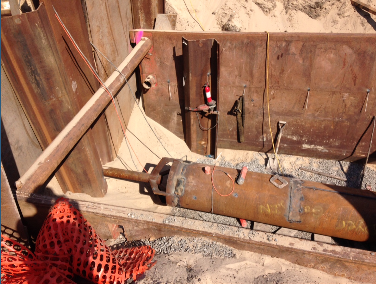
Pilot rod welded to steel casing
