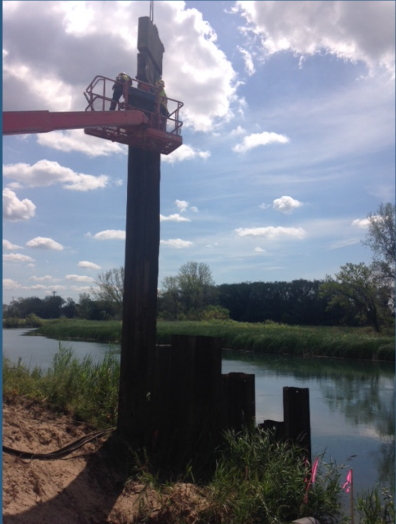
Installation of the sheet pile cofferdam
