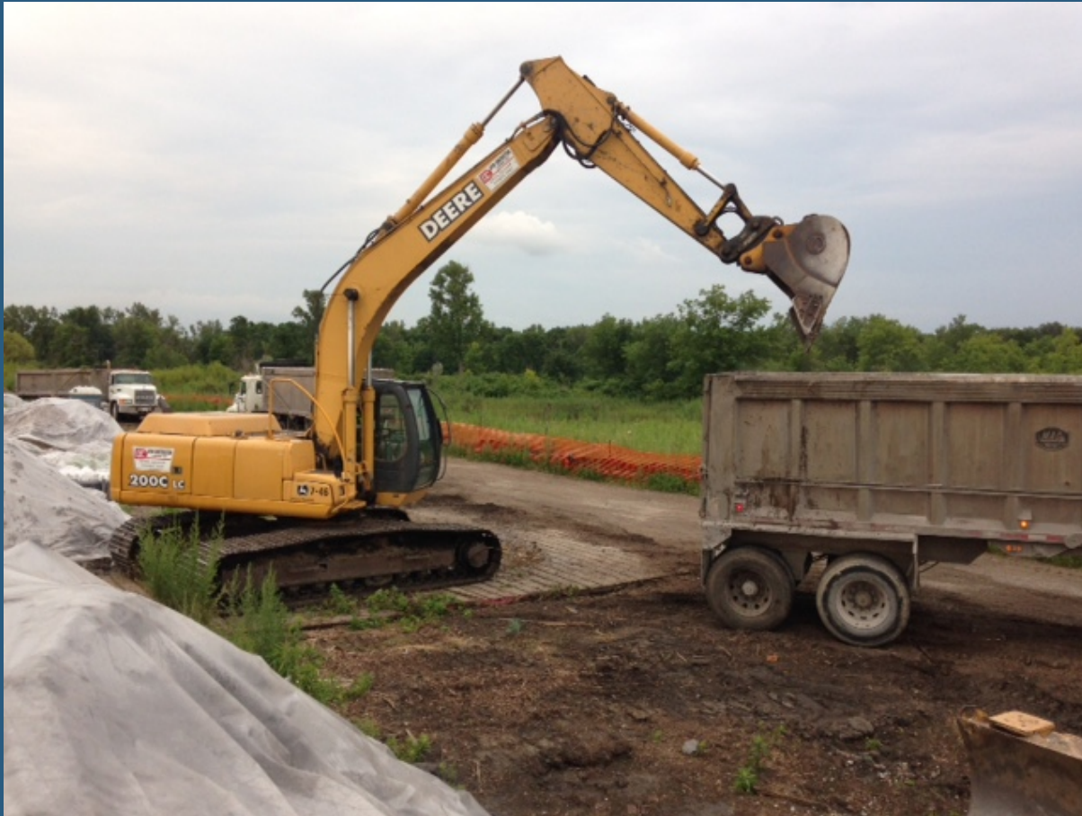
Loading and hauling off fly ash encountered during trenching
