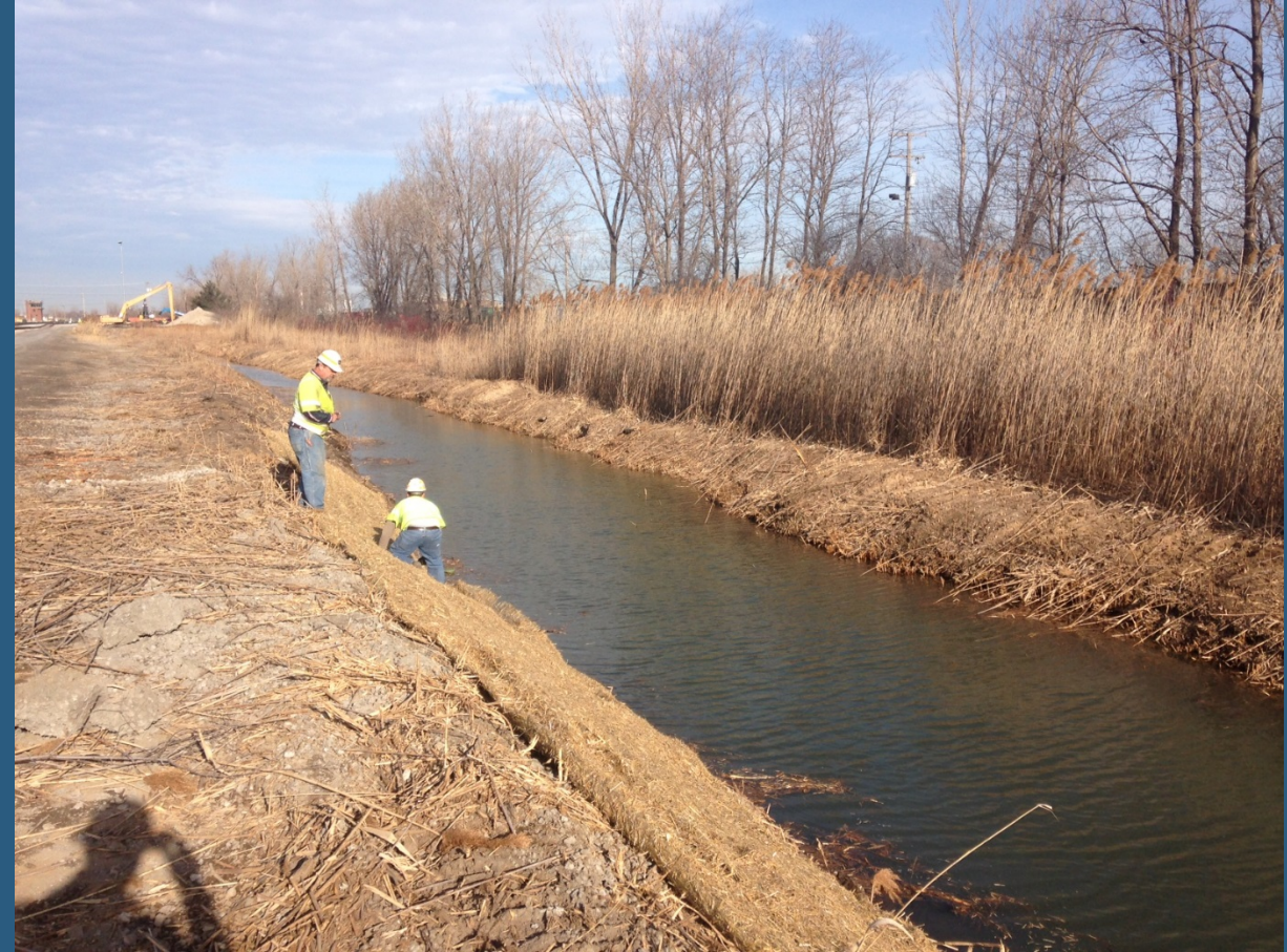
Installation of erosion control netting along Crowley Ditch slopes
