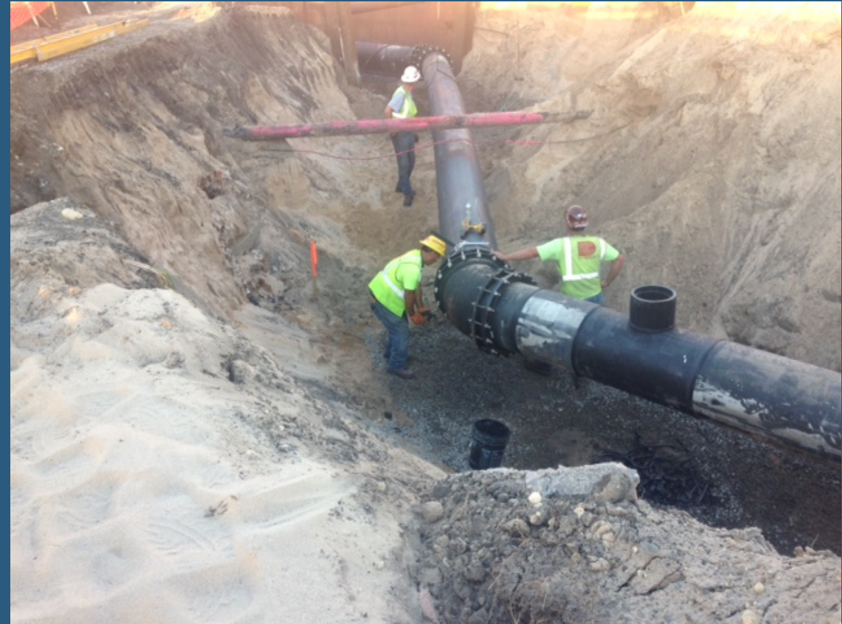
Open-cut installation: 45° bends, avoiding existing utilities, and tee-fitting for air-release valve
