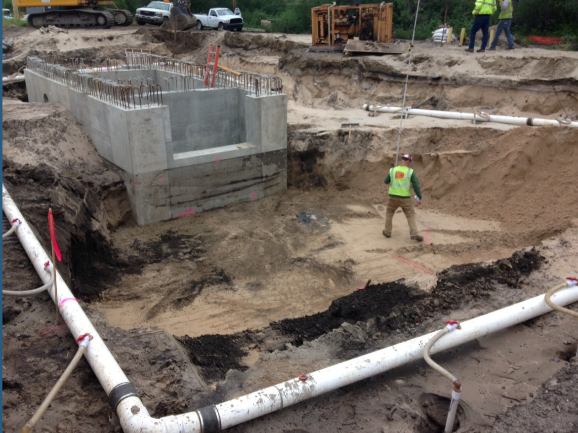
Wet well near complete; preparing subgrade for inlet channel
