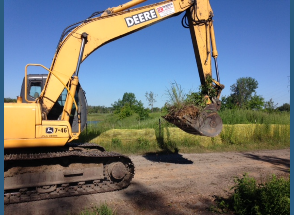
Excavate sensitive plants with root system intact
