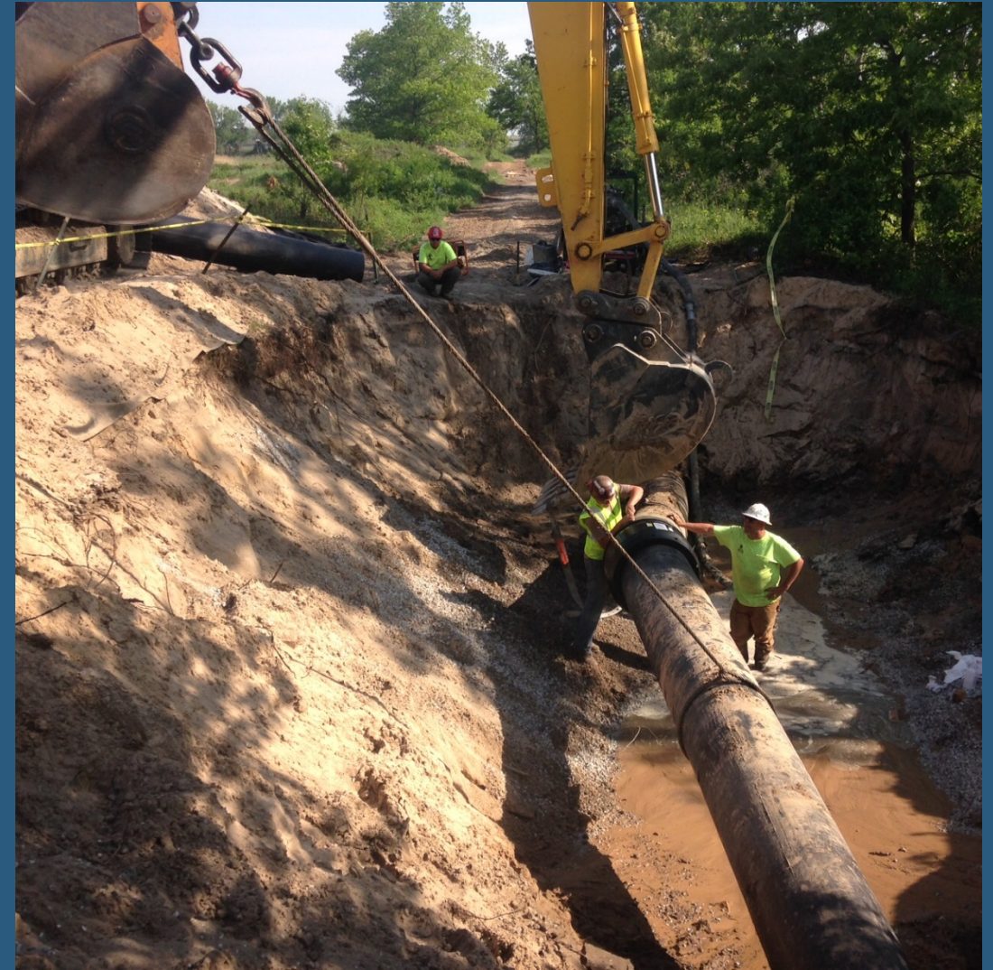
Using electro-fusion coupling to connect liner pipe at obstruction
