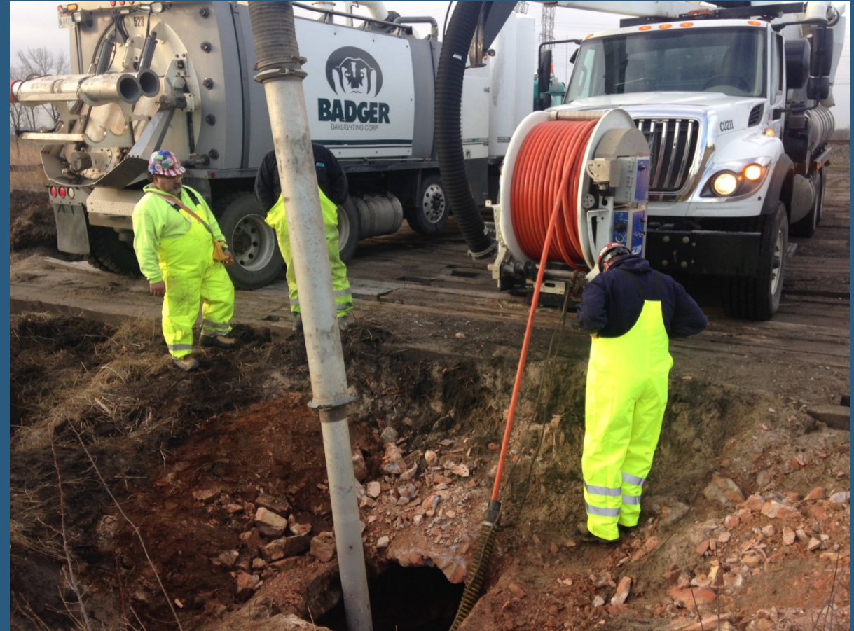
Using water jet and vacuum truck to clean brick sewer
