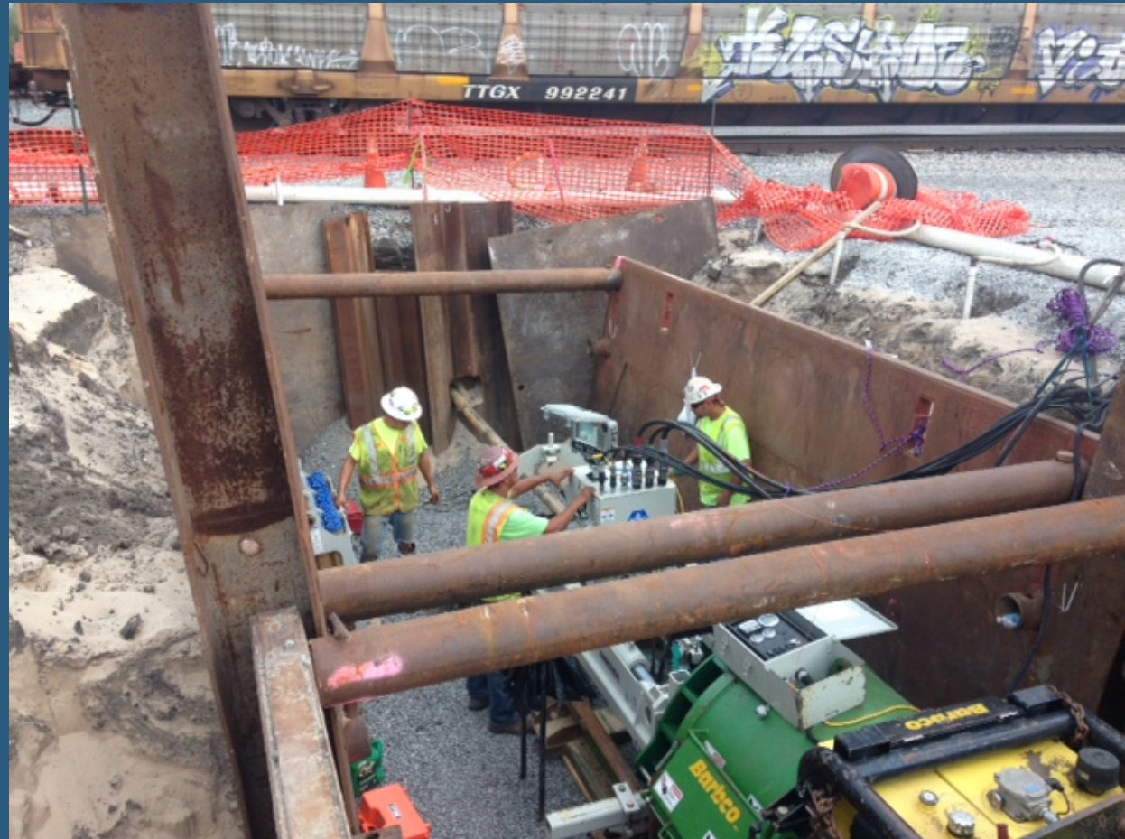
Pilot bore using the Ackerman Guided Boring System
