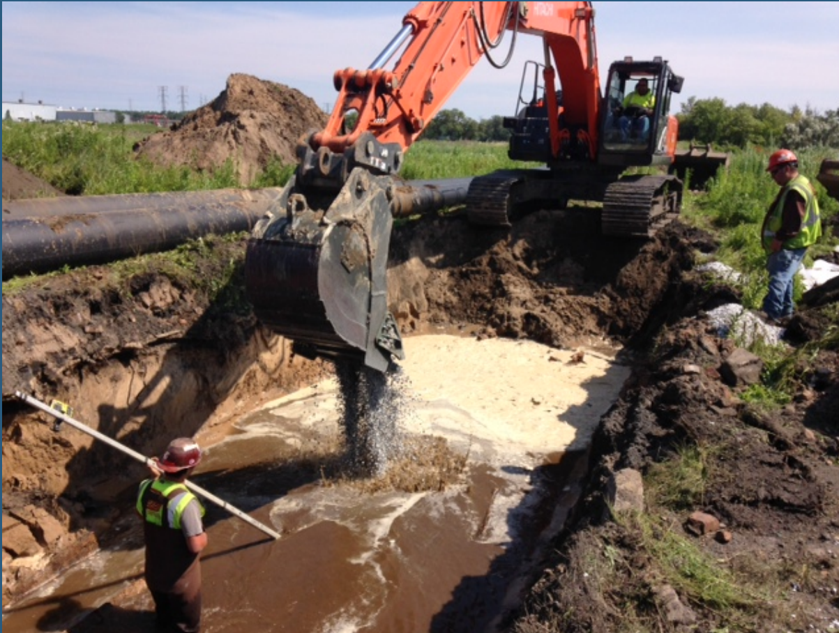
Placing and grading stone bedding at bottom of trench
