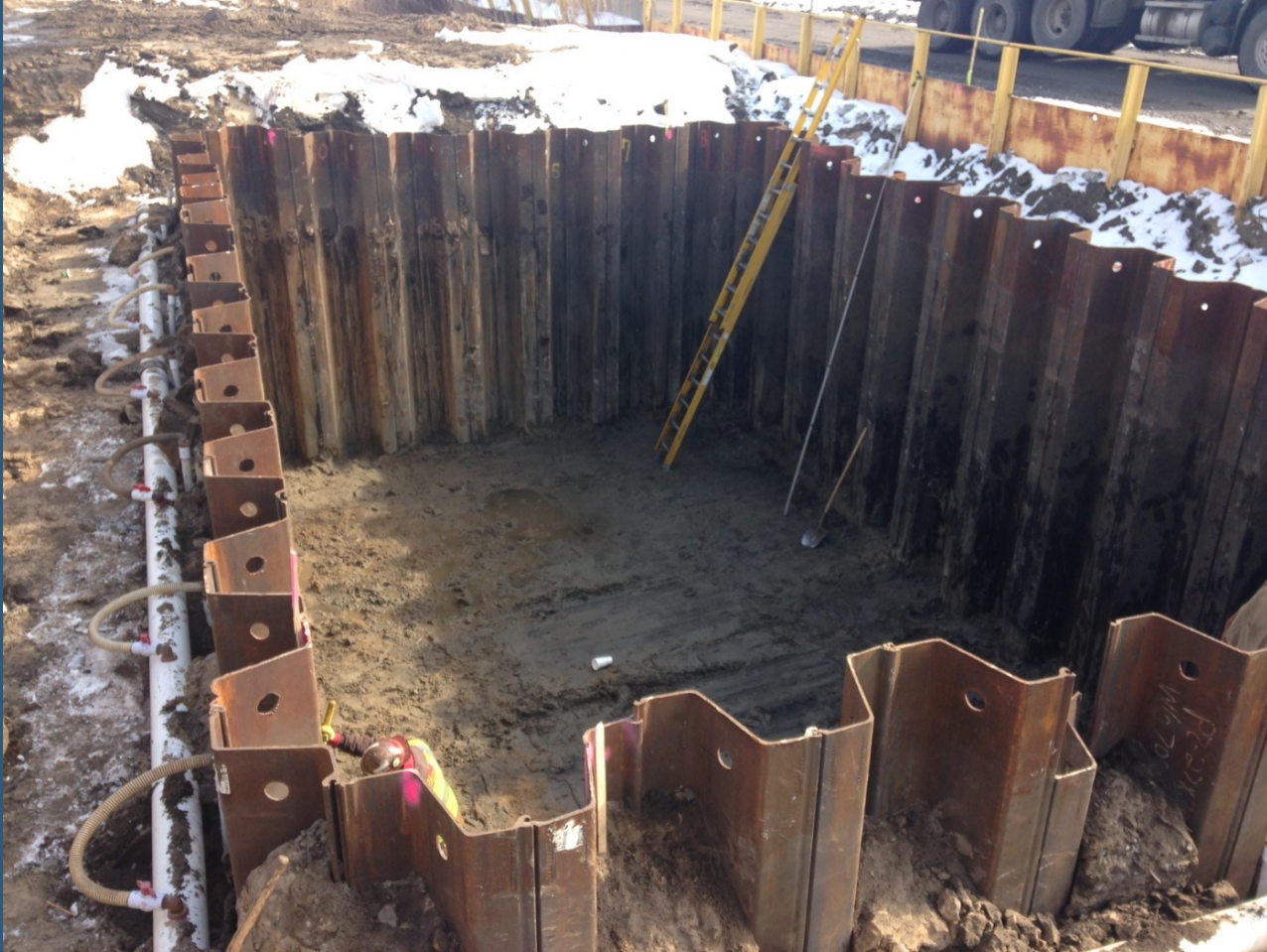
Sheet pile coffer dam and dewatering
