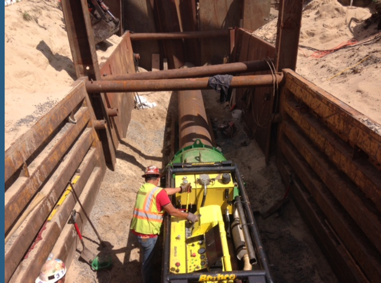
Jack & bore of the steel casing
