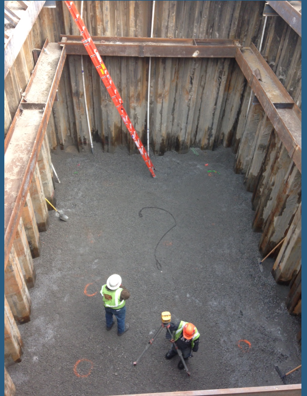
Completed excavation and subgrade preparation
