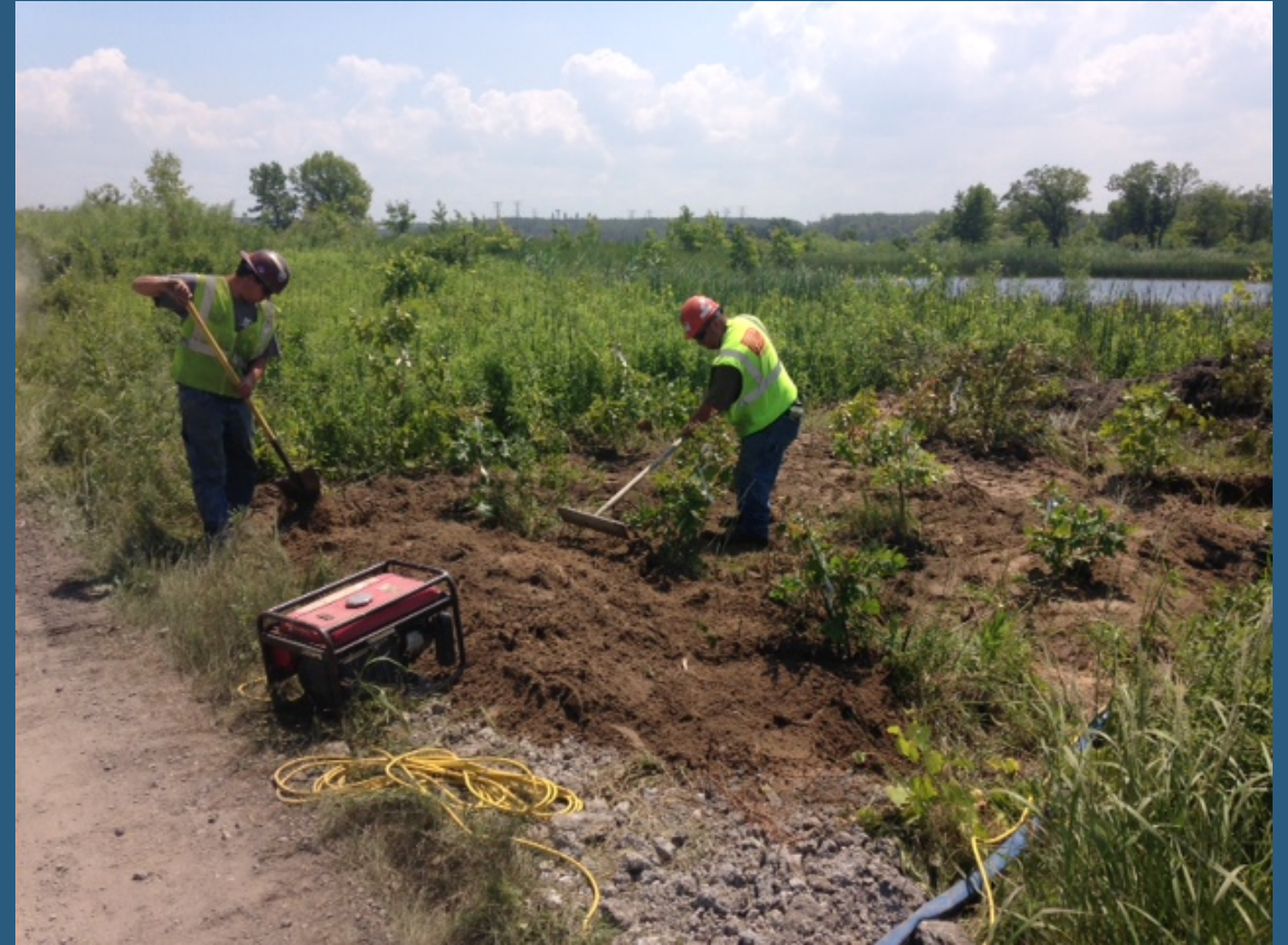
Placement, backfill, and watering of transplants
