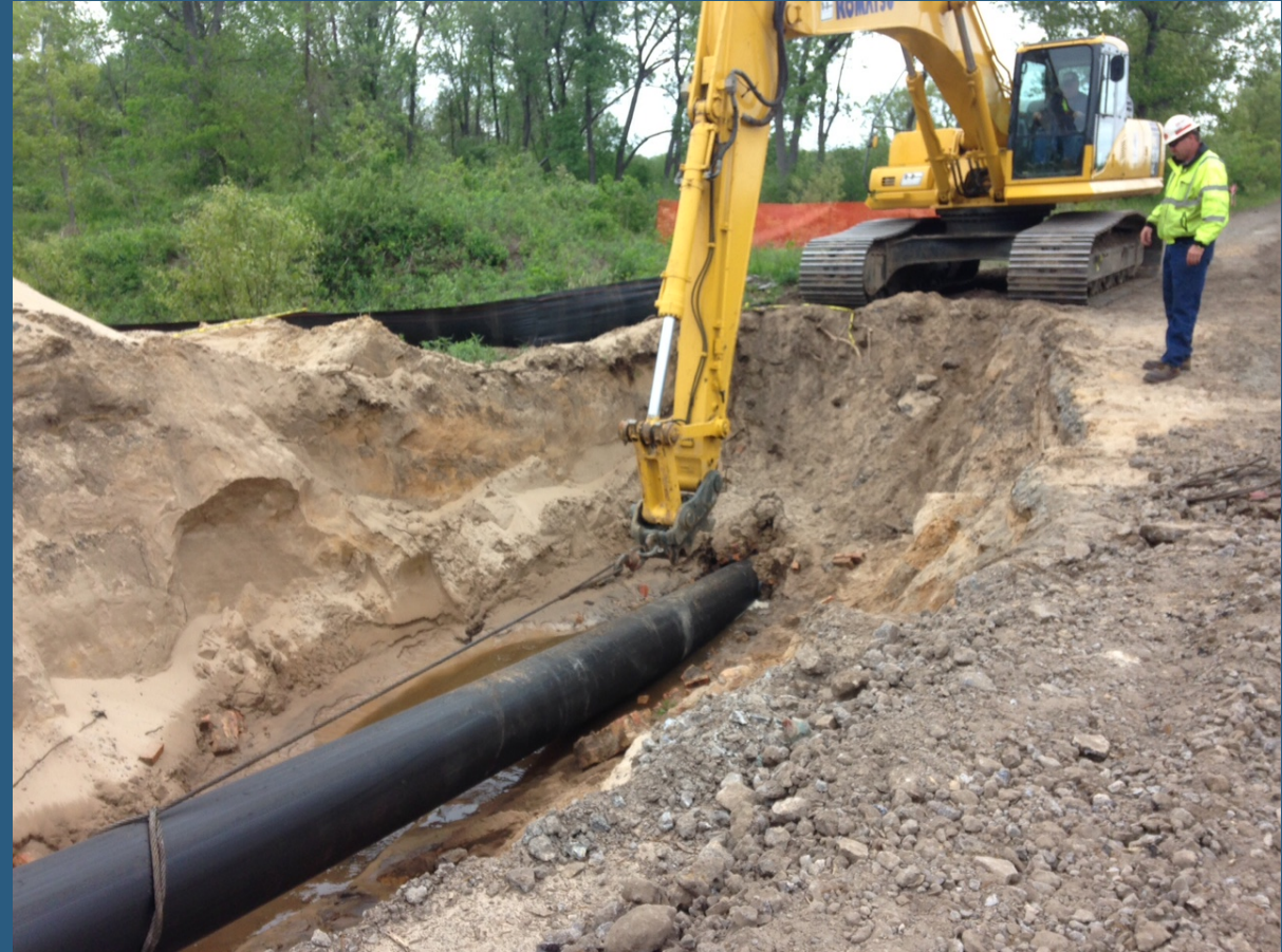
Assisting slip line with excavator to overcome underground debris
