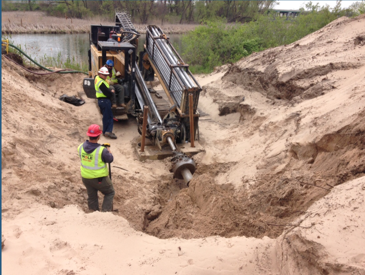
Slip line segment completed (~600')
