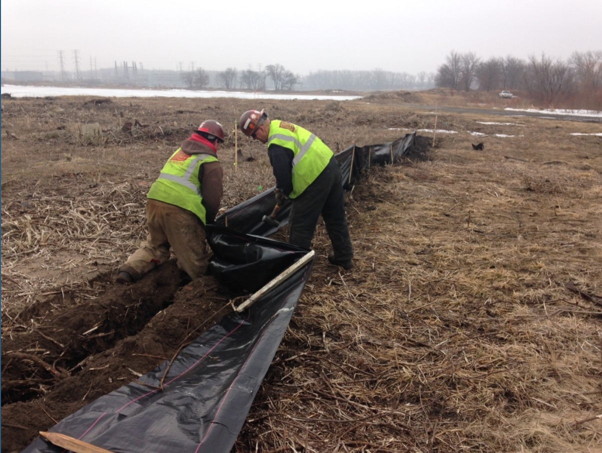
Installation of silt fence (following trench cut)
