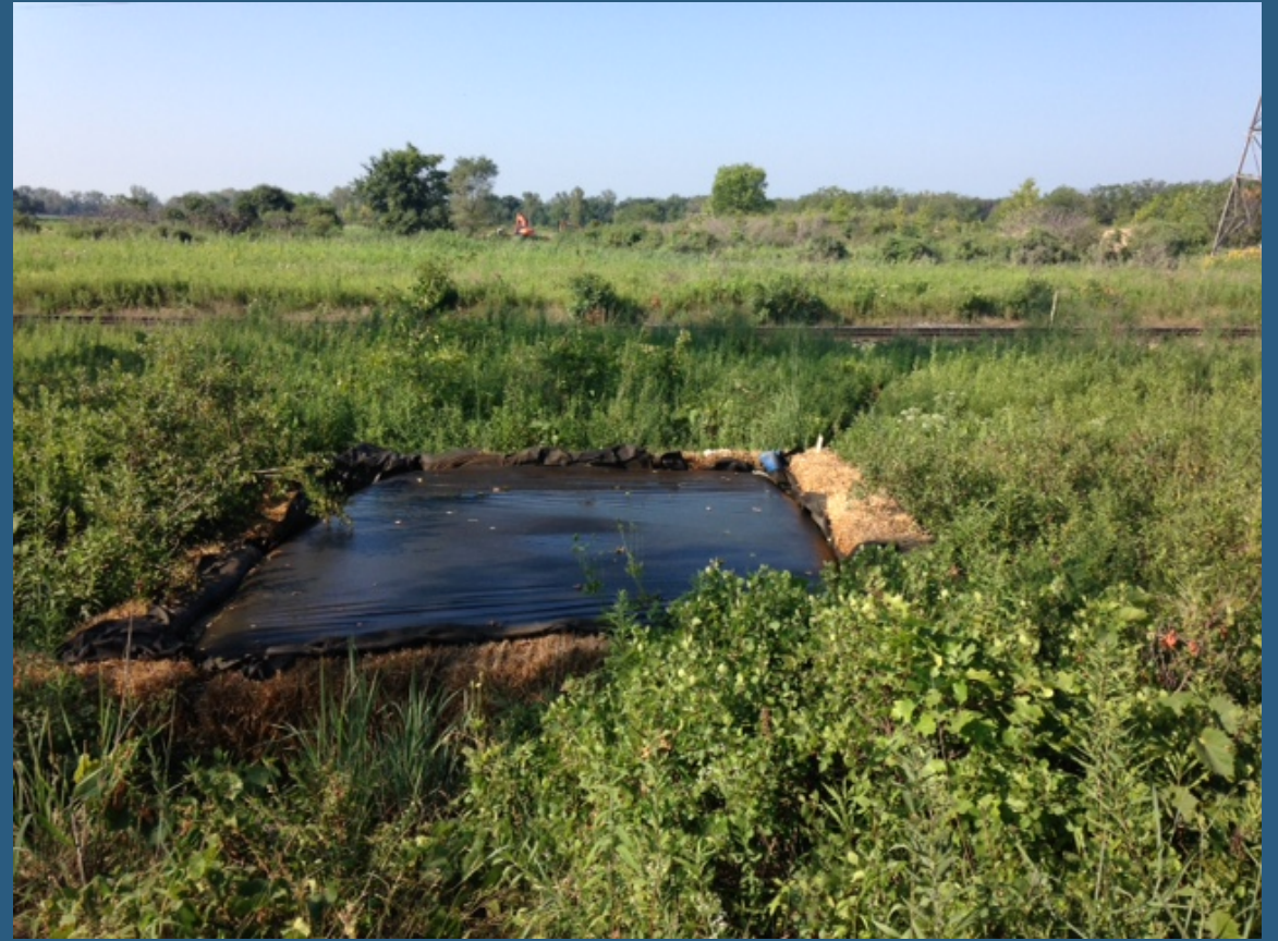
Dewatering filter basin
