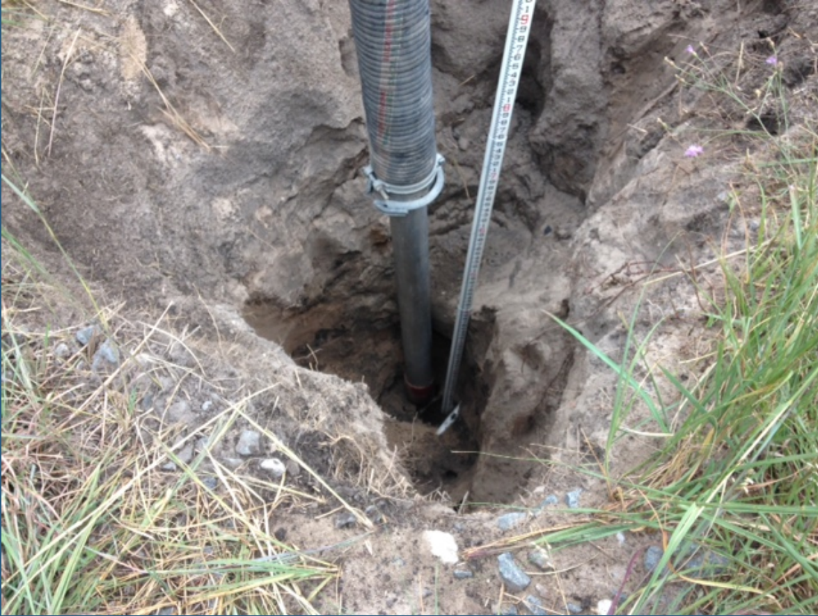
Potholing utilities with vacuum truck and surveying elevation
