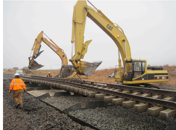
Figure 8 – Ballast Box Installation
