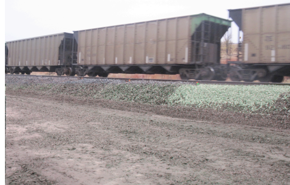
Figure 9 – Ballast Box Installation
