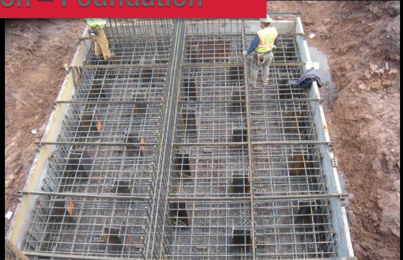
43,160 lbs reinforcement per abut.
