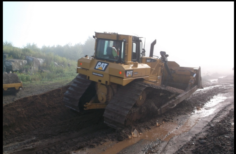
Removing Topsoil
