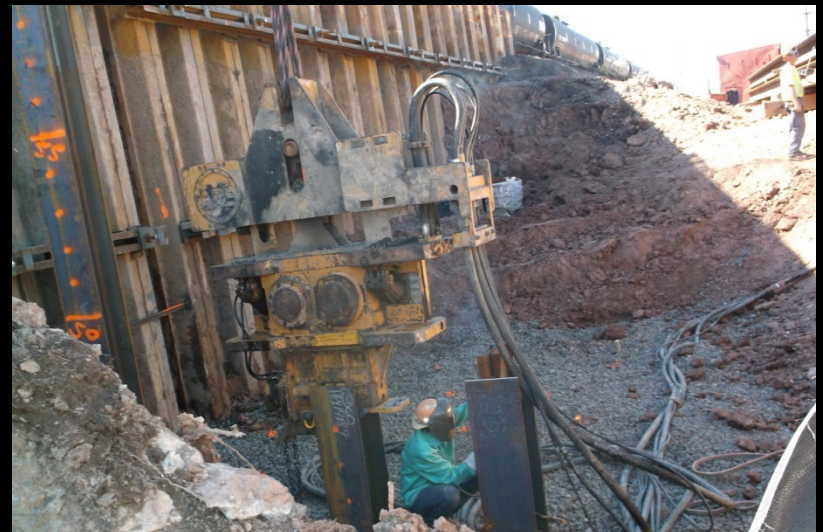
Shoring height = 24 ft
