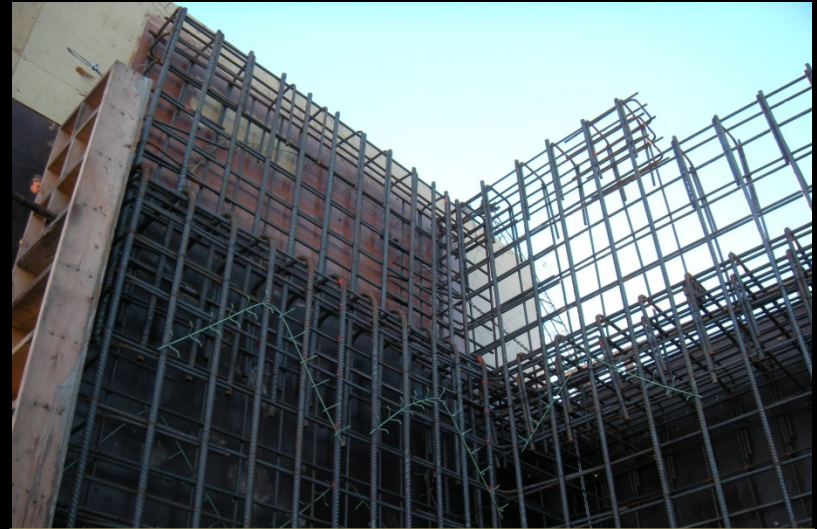
43,160 lbs reinforcement per abut.
