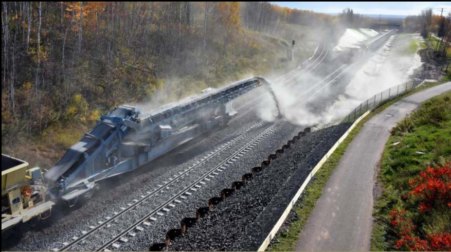
Grex ballast dumping train
