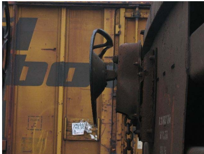
Figure 9.6 Brake wheel with insufficient clearance per CFR Part 231
