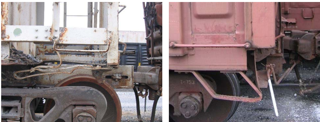
Figure 9.18 Sill step deformation showing an FRA defect (left) and significant deformation (right)
