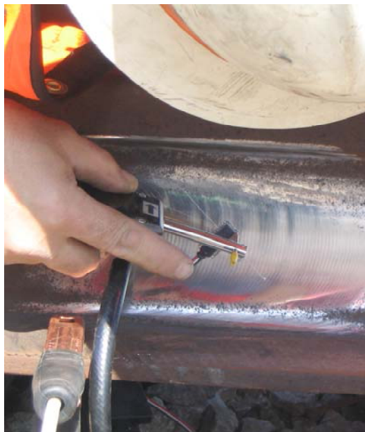
Figure 3.1 Spot-Welded Strain Gauge Installation
