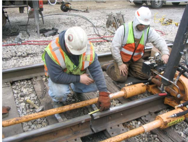
Figure 2.4 Rail Restressing
