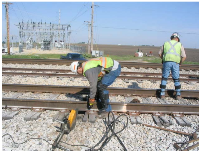
Figure 2.3 Rail Destressing
