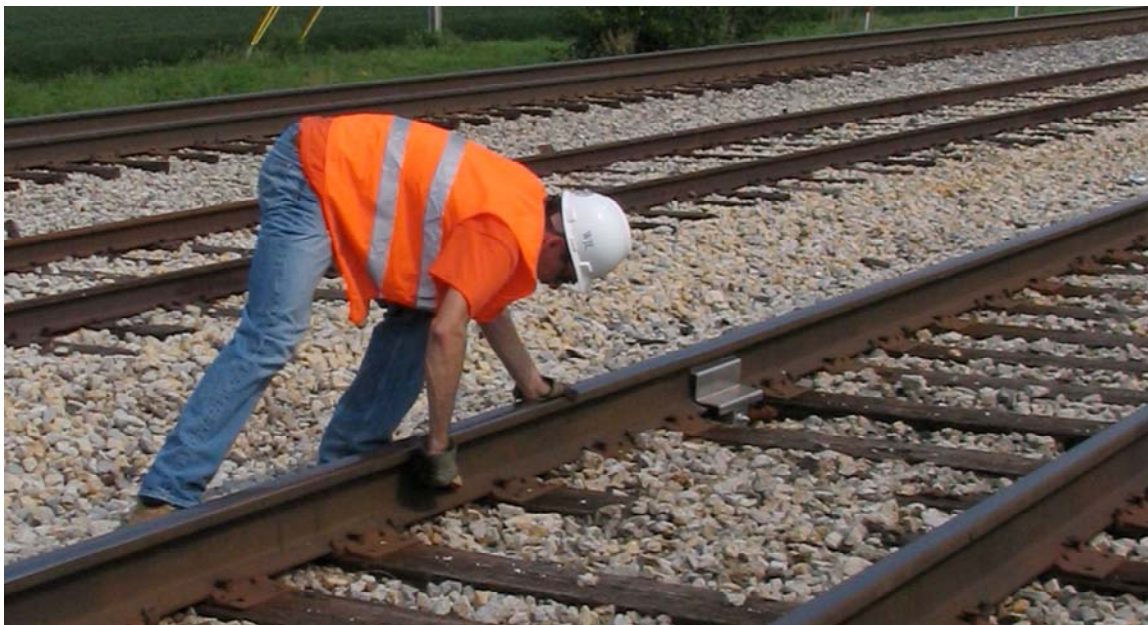
Figure 9.16 Preparing the Rail Surface
