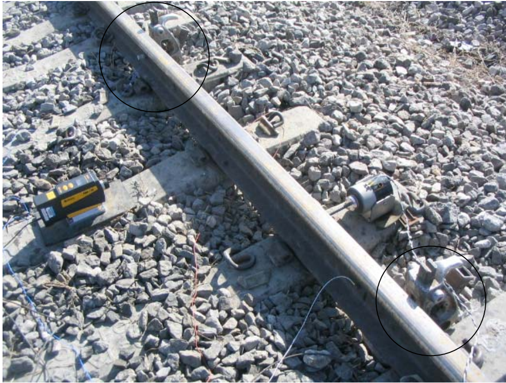
Figure 9.13 Track Jacks on Concrete Tie Track
