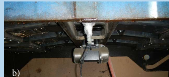
Plant B vibrator under forms
