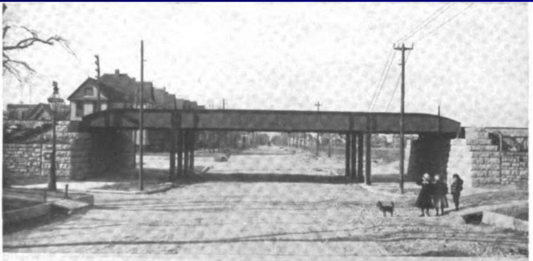
FIG. 451. BRIDGE AT MONTROSE AVE., 80 FT. BETWEEN ABUTMENTS, POSTS ON CURB LINE.
