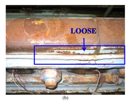
Figure 1: Classifications of damage to the top edge of the insulator layer. (a) Loose and Missing. (b) Loose only.
