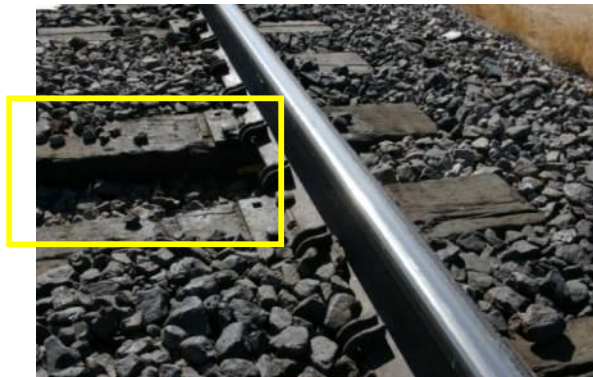
Figure 3.3: Example of Low Crib Ballast between a Pair of Ties
