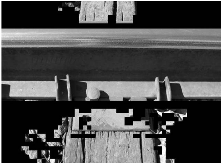
Figure 8.3: Isolated Non-Ballast Objects Including the Rail, Tie Plate, Tie, and Anchors
