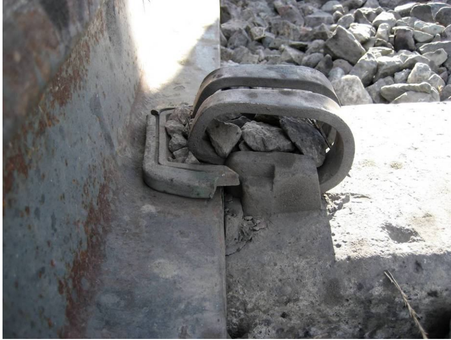
Figure 7.1: Potential Camera View for Machine-vision Inspection of Concrete Tie Rail Seat Abrasion
