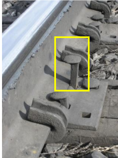
Figure 3.7: Example of a Raised Cut Spike
