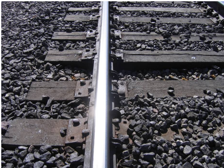
Figure 6.7: Image from Over-the-rail View Recorded at TTC's FAST
