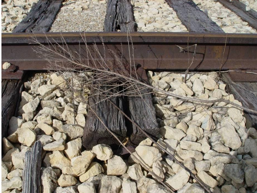
Figure 7.4: View of Spikes with Obstructions on a Local Low-density Rail Line
