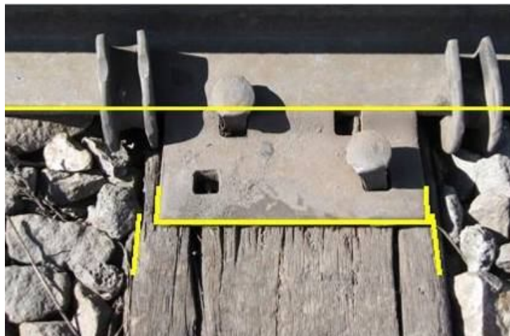
Figure 8.4: Delineated Rail, Tie Plate, and Tie
