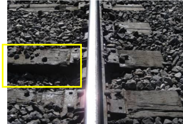
Figure 3.5: Another Example of Low Crib Ballast
