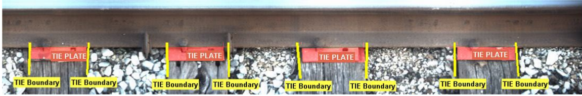
Figure 8.8: Tie and Tie Plate Delineation on Test Panorama
