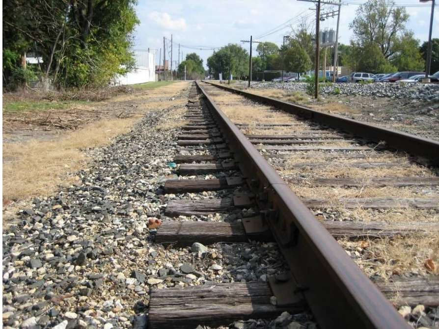
Figure 7.2: Initial Camera View for Ballast Shoulder Profile Inspection
