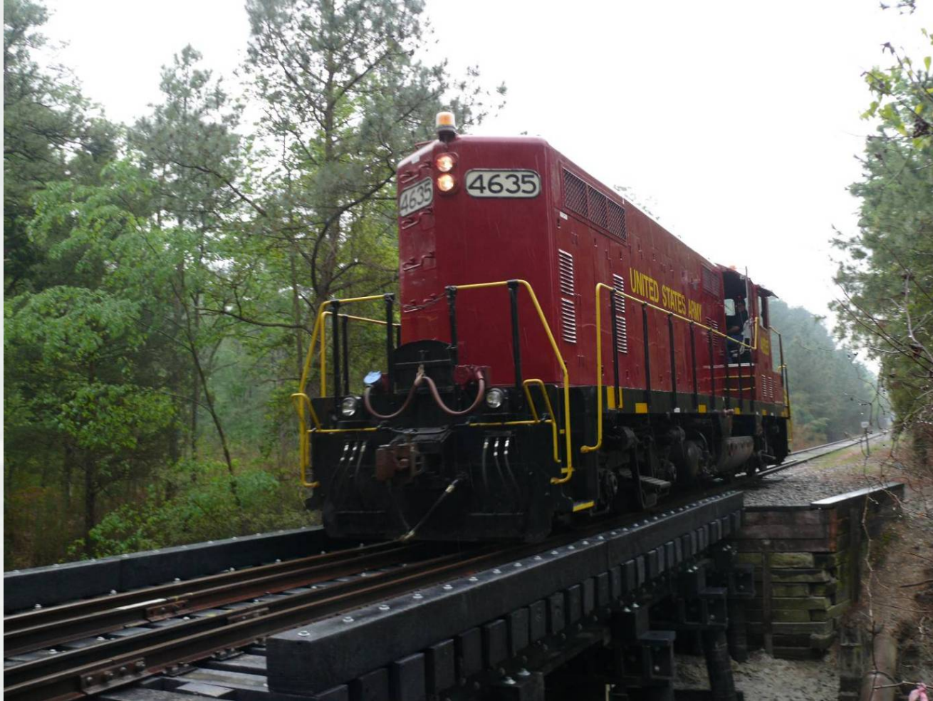
All plastic composite RR bridge at Fort Eustis, VA
