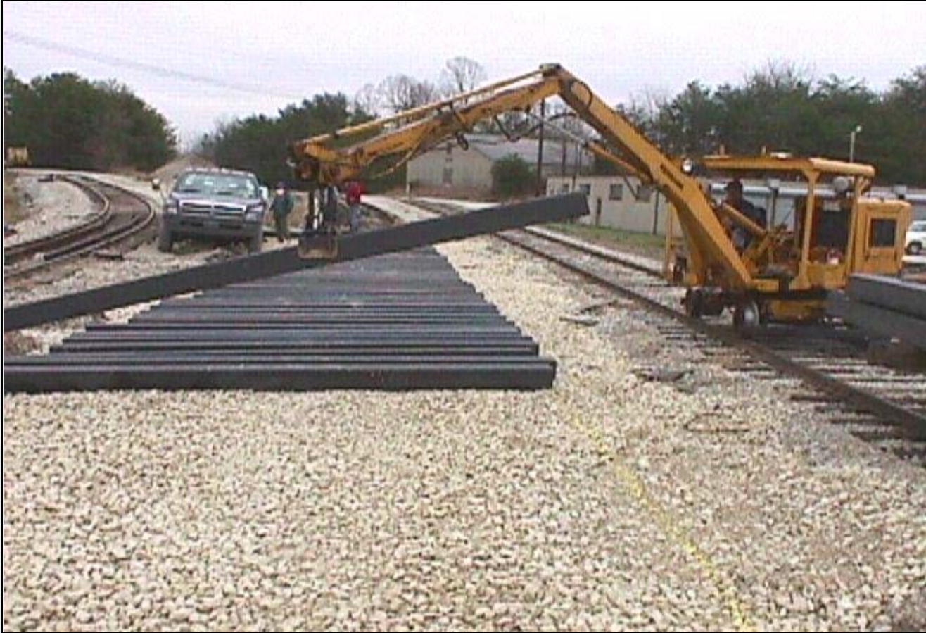
Laying Out SwitchTies
