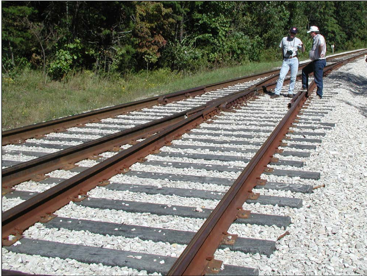
Second Plastic Tie Turnout Completed June 2002
