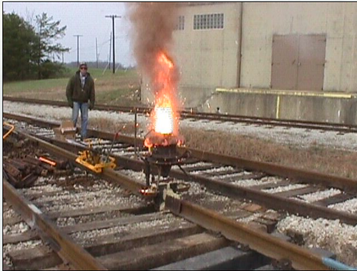
Thermite Welding
