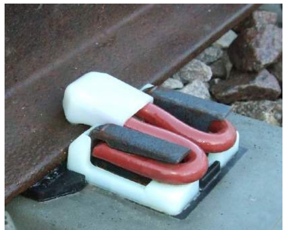
Figure 1.4 Most common clip-type fastening systems found in North America (Adapted from CEB FIP 1987 and Kerr 2003)
