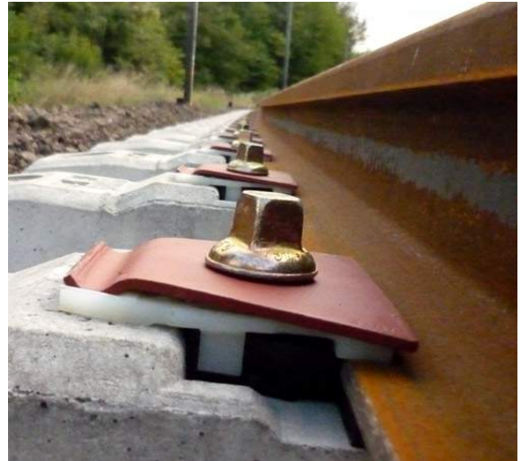
Figure 1.3 Elastic fastenings - Screw systems (Adapted from CEB FIP 1987)
