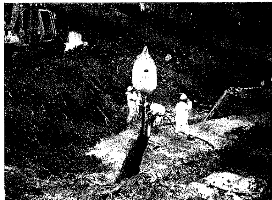
Figure 12 Installation of Bentonite Containment Wall (BCW)
