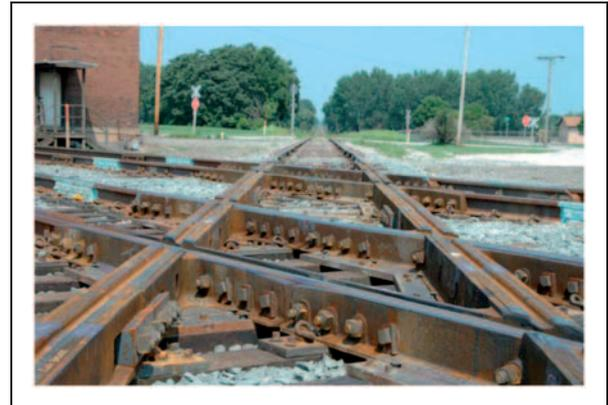
**Figure 2.** Example of an OWLS partial flange bearing line. Reproduced with permission from the American Railway Engineering and Maintenance-of-way Association.
