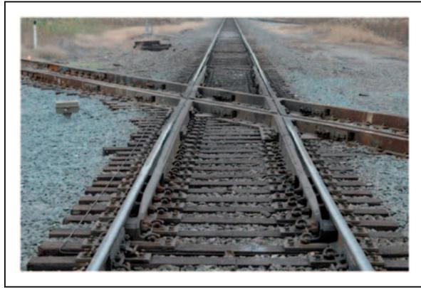
**Figure 1.** Example of a FBF diamond. Reproduced with permission from the American Railway Engineering and Maintenance-of-way Association.
