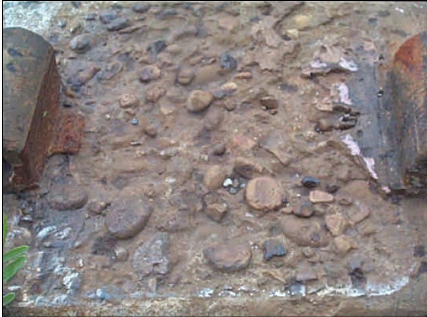
**FIGURE 3. Service example of rail seat deterioration suggesting erosion of the cement paste (5)**
