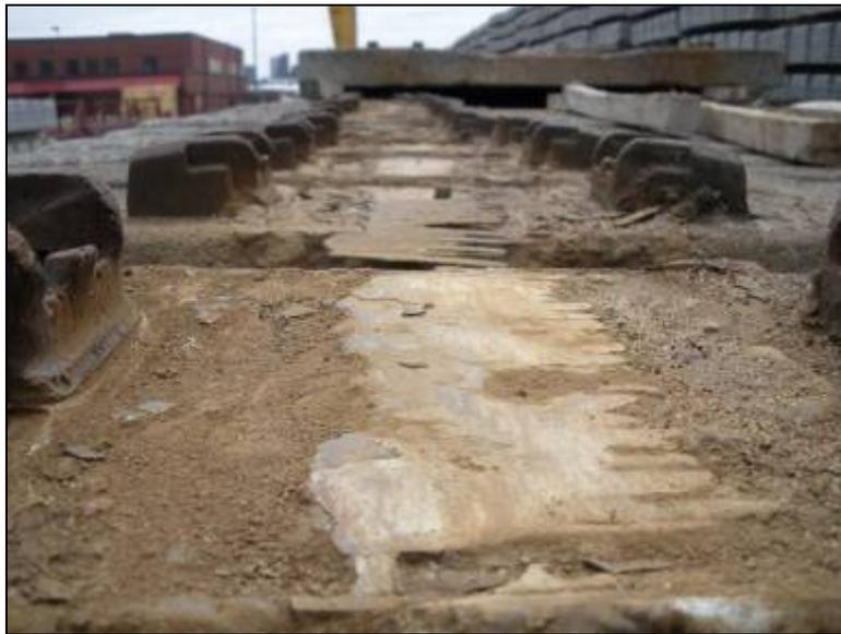
**FIGURE 2. Service example of rail seat deterioration suggesting loosened fastening components**
