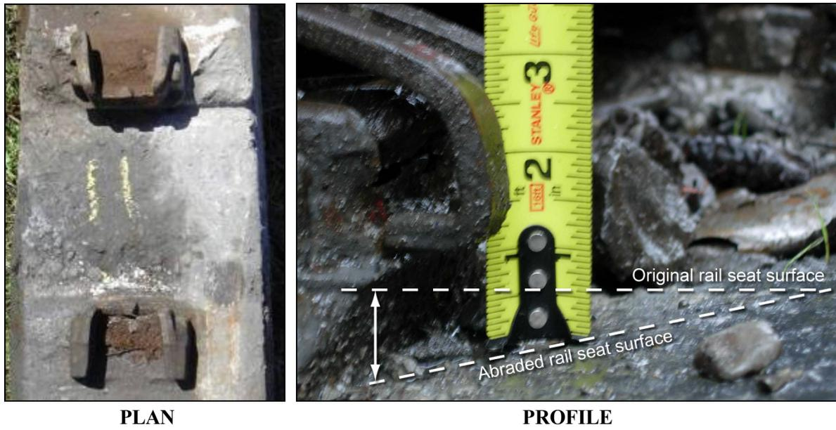
**FIGURE 1. Service examples of rail seat deterioration suggesting lateral forces on a curved section of track (4)**
