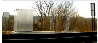
Figure 5: Southern view of the Sibley machine vision installation, showing from left to right, the AEI reader, equipment bungalow, camera, communication tower and exposure target
