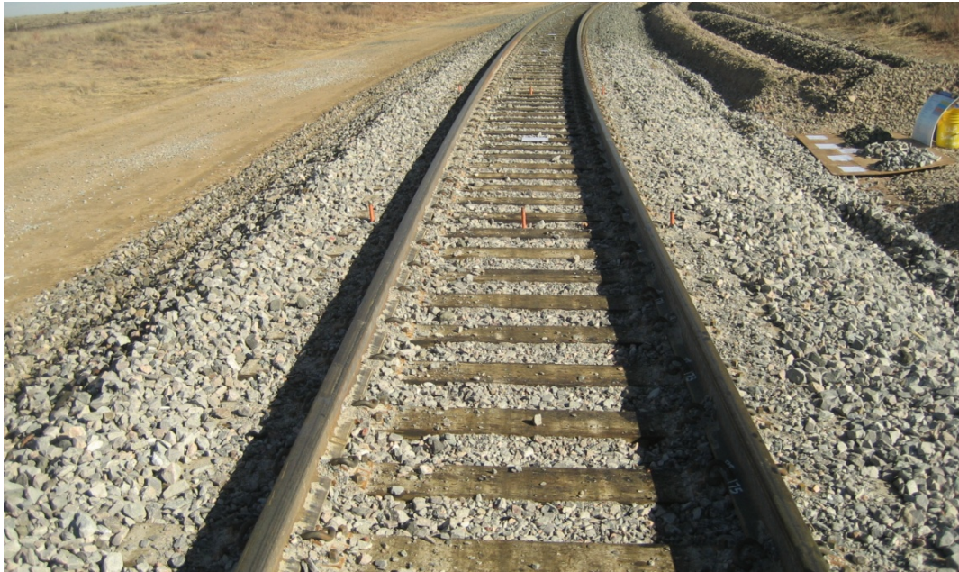
Figure 5 Photo Showing the Final Constructed Ballast Test Section
