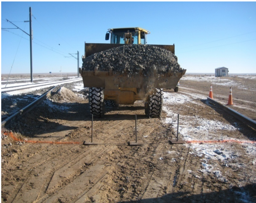
Figure 4 Photo Showing Settlement Plate Installations
