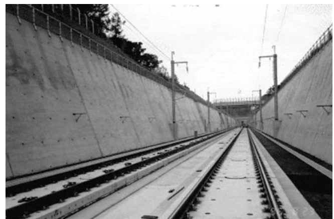
Fig. 10 RCRS laid on cutting in Hokuriku Shinkansen line
