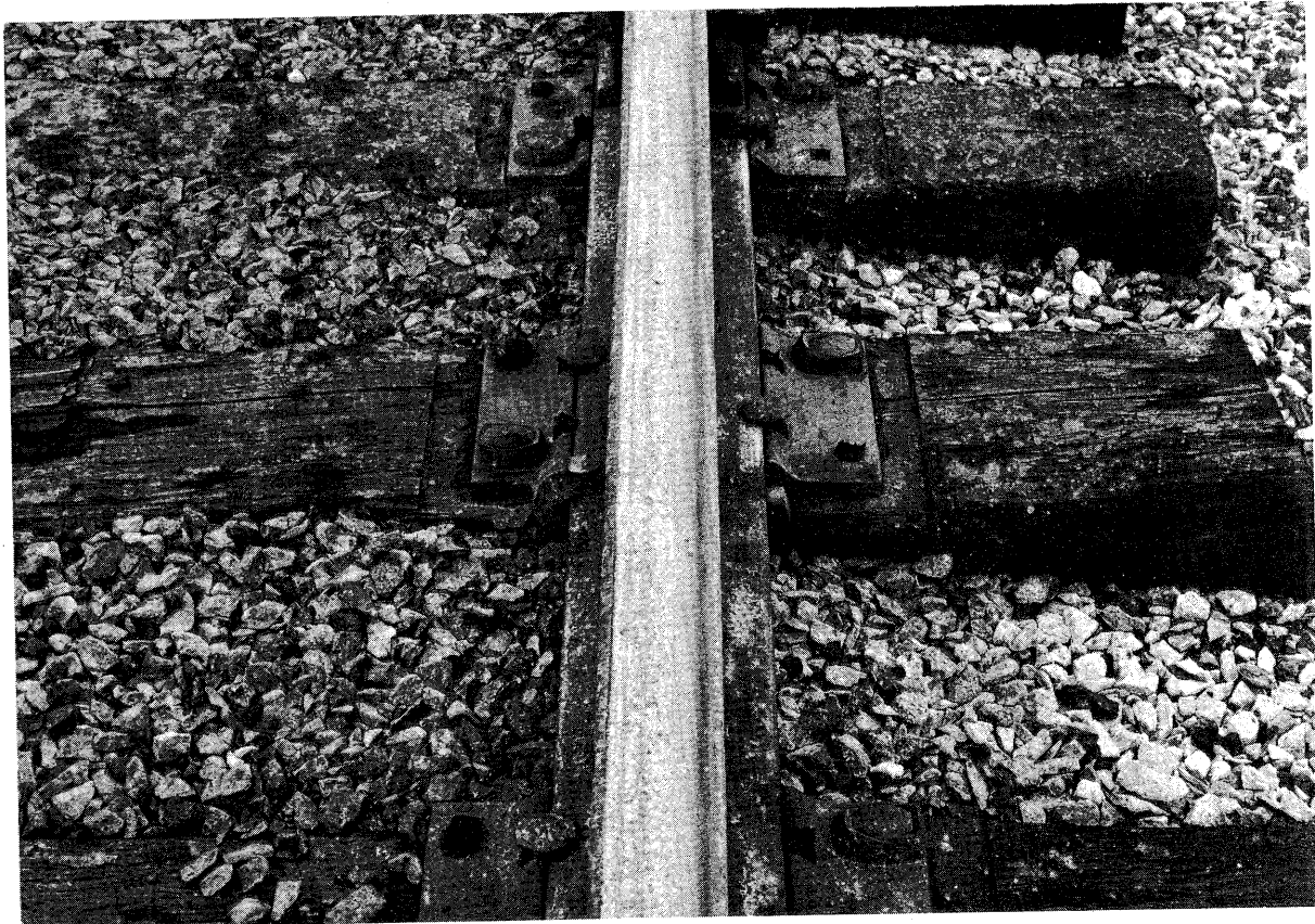
Fig. 9--Section 9, 2 Rubber Anchor Spike Cushions on North 10 Ties.
