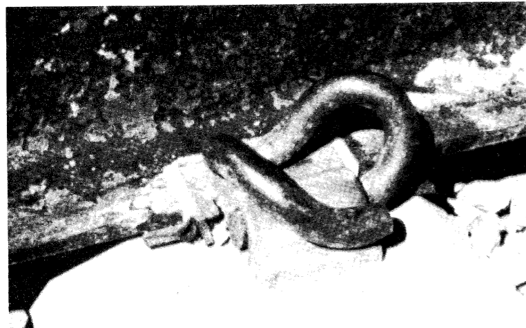
Type F-1 threadless elastic clip with external insulator. (Type F-2 uses the same clip with insulation bonded inside shoulder.)
