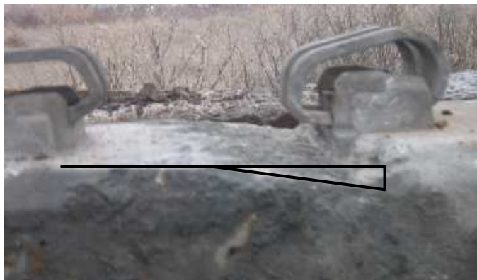
Figure 1. Triangular abrasion pattern in a concrete tie with black lines outlining a triangular pressure distribution assumed for this analysis.
