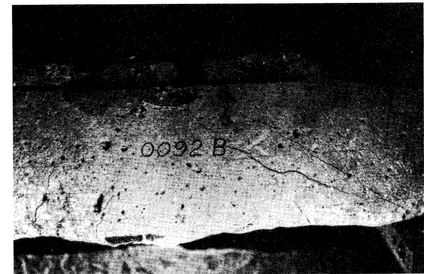
After ultimate load
