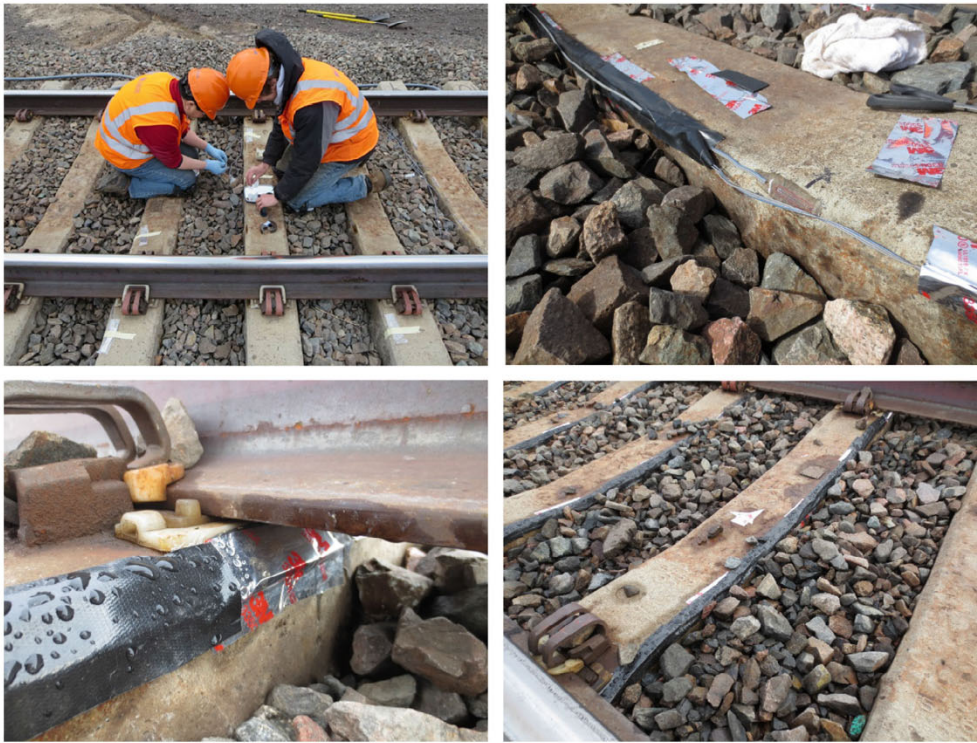
Fig. 5. Images of sleepers instrumented with concrete surface strain gauges at a heavy-haul freight railroad field experimentation location.
