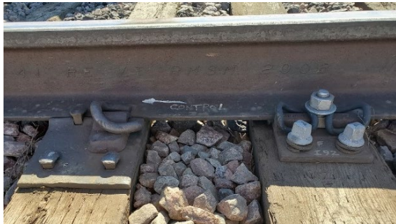
Figure 1. Transition between control fastener (left) and alternative fastener (right) at TTC's FAST
