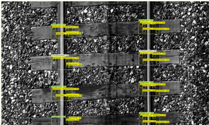
Figure 4. Two missing spikes detected since the surrounding crossie plates have five spikes.
