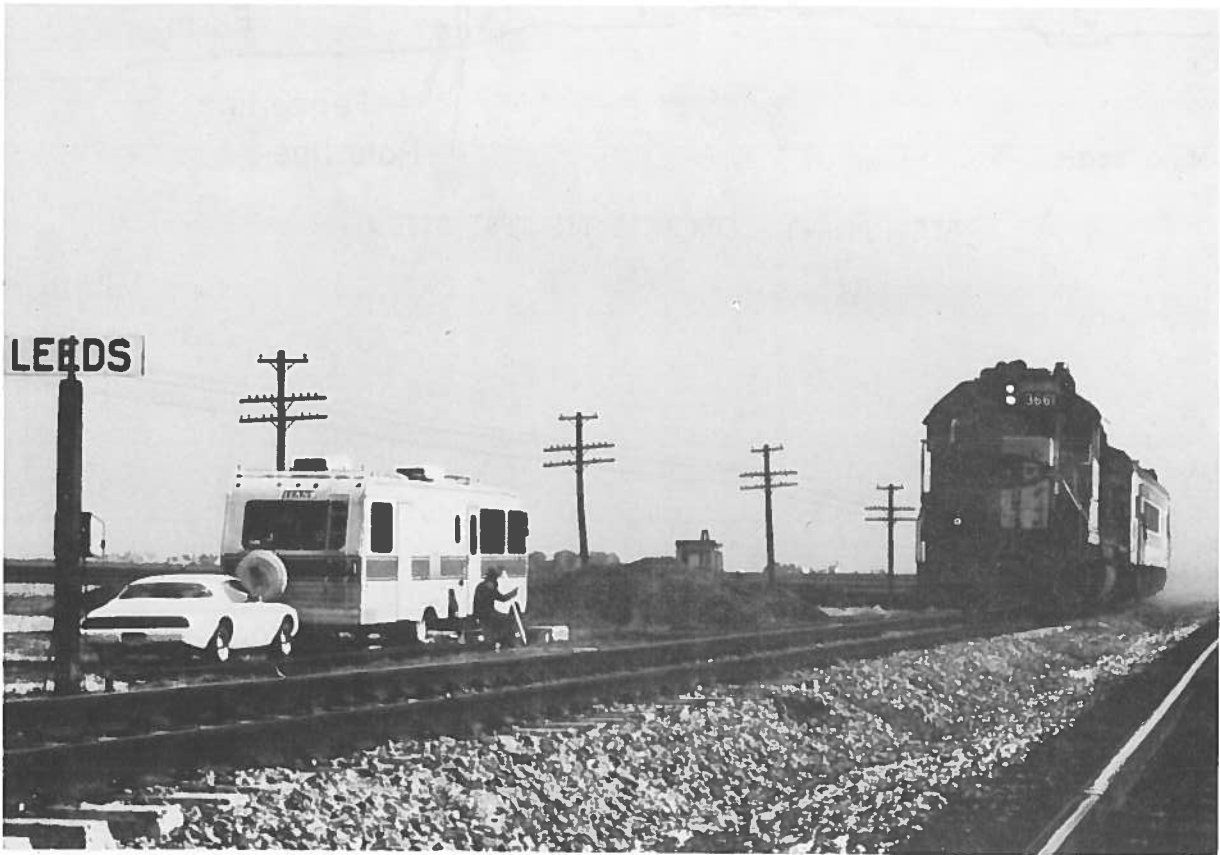
FIGURE 4. AT&SF CONCRETE TIE TEST SITE, STREATOR (LEEDS), ILL., WITH WESTBOUND GEOMETRY CAR
