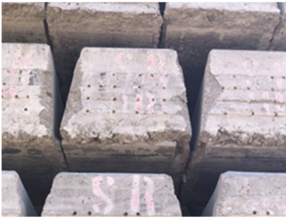
Fig. 1. Concrete crosstie with under tie pads (UTPs) [5].
