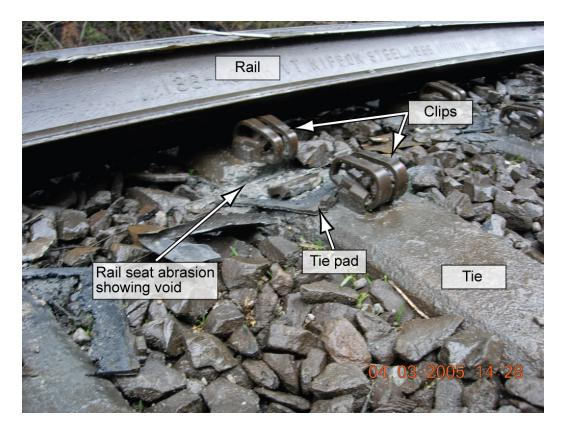
Figure 4. Rail rollover and rail seat abrasion at derailment site.
