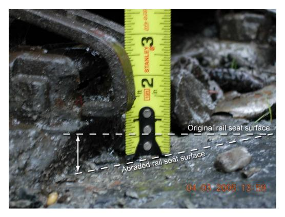
Figure 5. Concrete crosstie abrasion of about 1 inch at derailment site.
