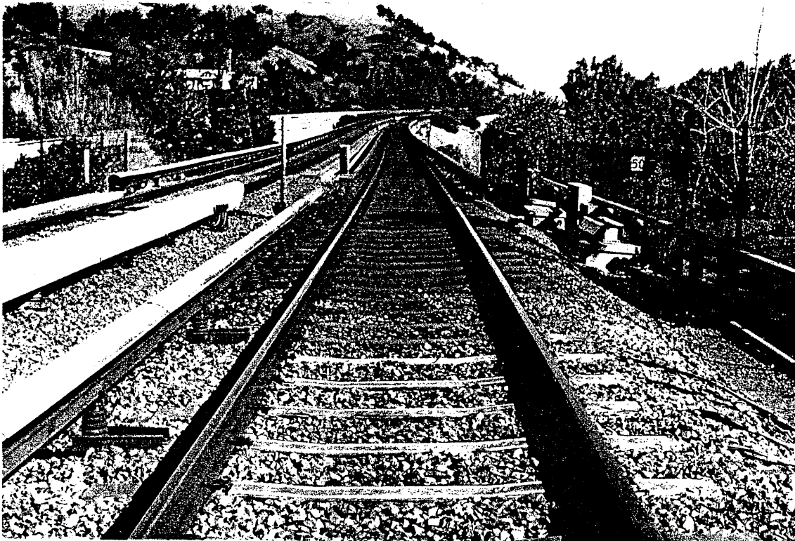
Figure 2 Test Site - Looking East
